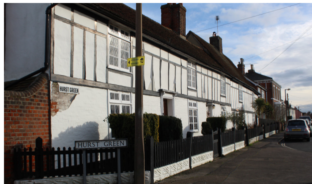
Figure 27 Grade II Listed 29 and 30 Hurst Green
