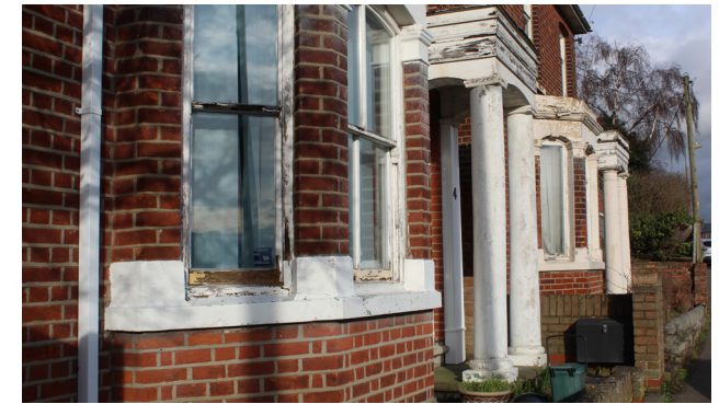
Figure 25 Architectural detailing of houses on Hurst Green
