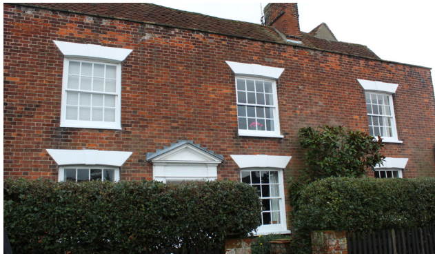
Figure 70 Grade II Listed 42 Queen Street
