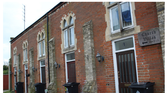
Figure 79 Former Congregational Chapel
