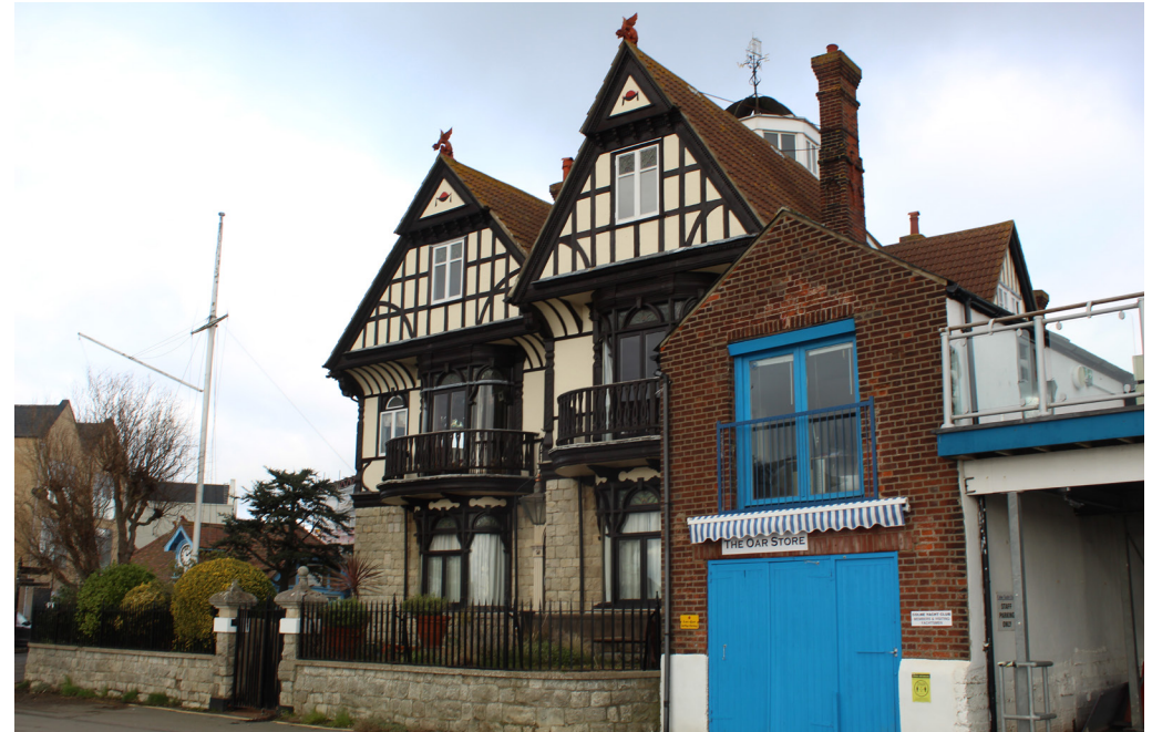
Figure 38 The Waterfront Character Area (Oar Store and former Anchor Hotel)
