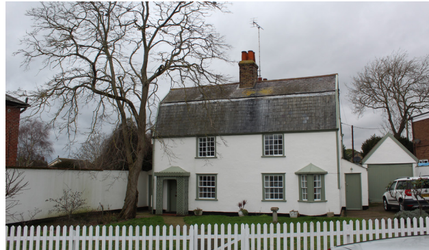
Figure 65 Grade II Listed Lower Green Cottage
