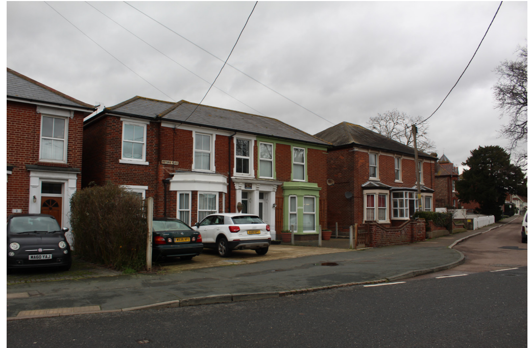
Figure 56 Station Road Character Area
